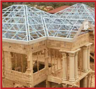
STEEL ROOF TRUSSES
